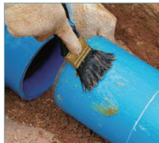
3. Apply lubricant on spigot
