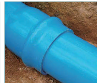
4. Insert the pipe until the white line
