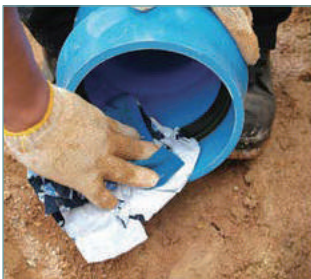
1. Clean dirt and grit from socket
