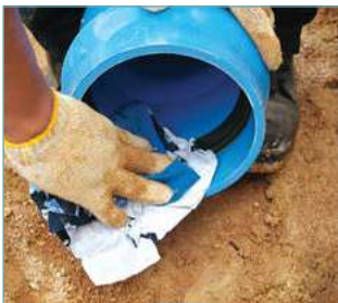
1. Clean dirt and grit from socket
