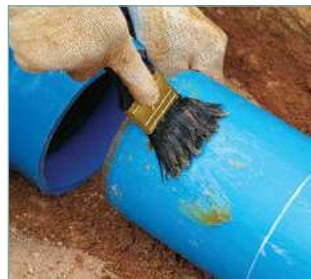
3. Apply lubricant on spigot
