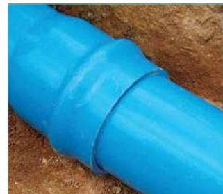
4. Insert the pipe until the white line
