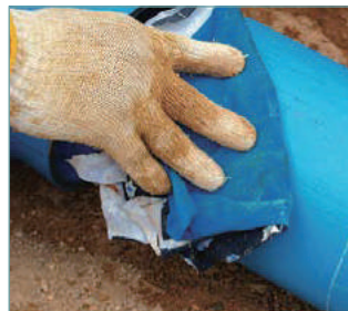
2. Clean the exterior of the pipe before applying the lubricant
