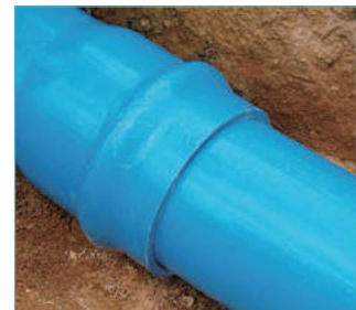
4. Insert the pipe until the white line
