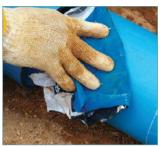
Clean the exterior of the pipe before applying the lubricant
